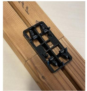
In the case of the installation of boards with Grad clips, it is necessary at the joint of the end pin, to fix the boards with Grad clips to prevent the boards from shifting sideways as a
